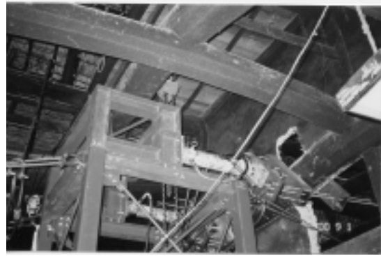
Photo1 inside establishment type load test device
