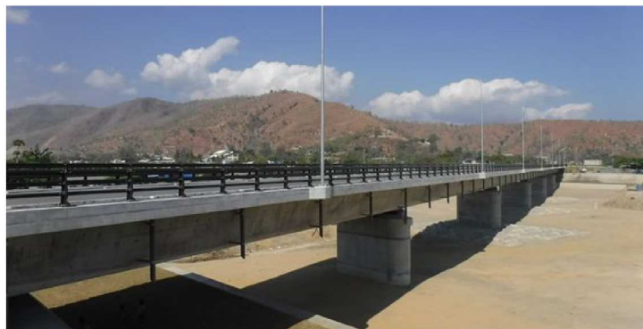
Figure 4. 10 Real bridge model
