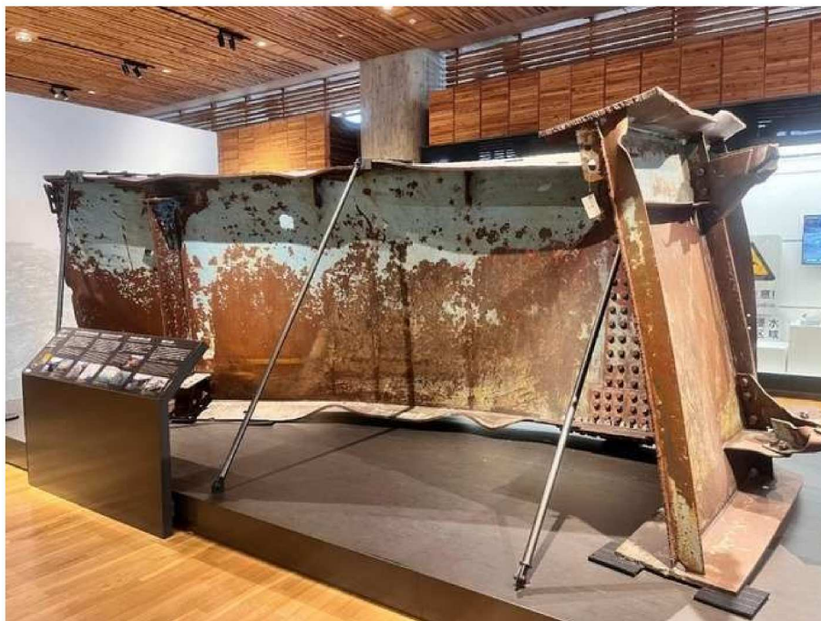
Figure. Kesen Ohashi Bridge Part Damaged by Tsunami Disaster, Iwate Tsunami Museum, Source: Author (2024).
