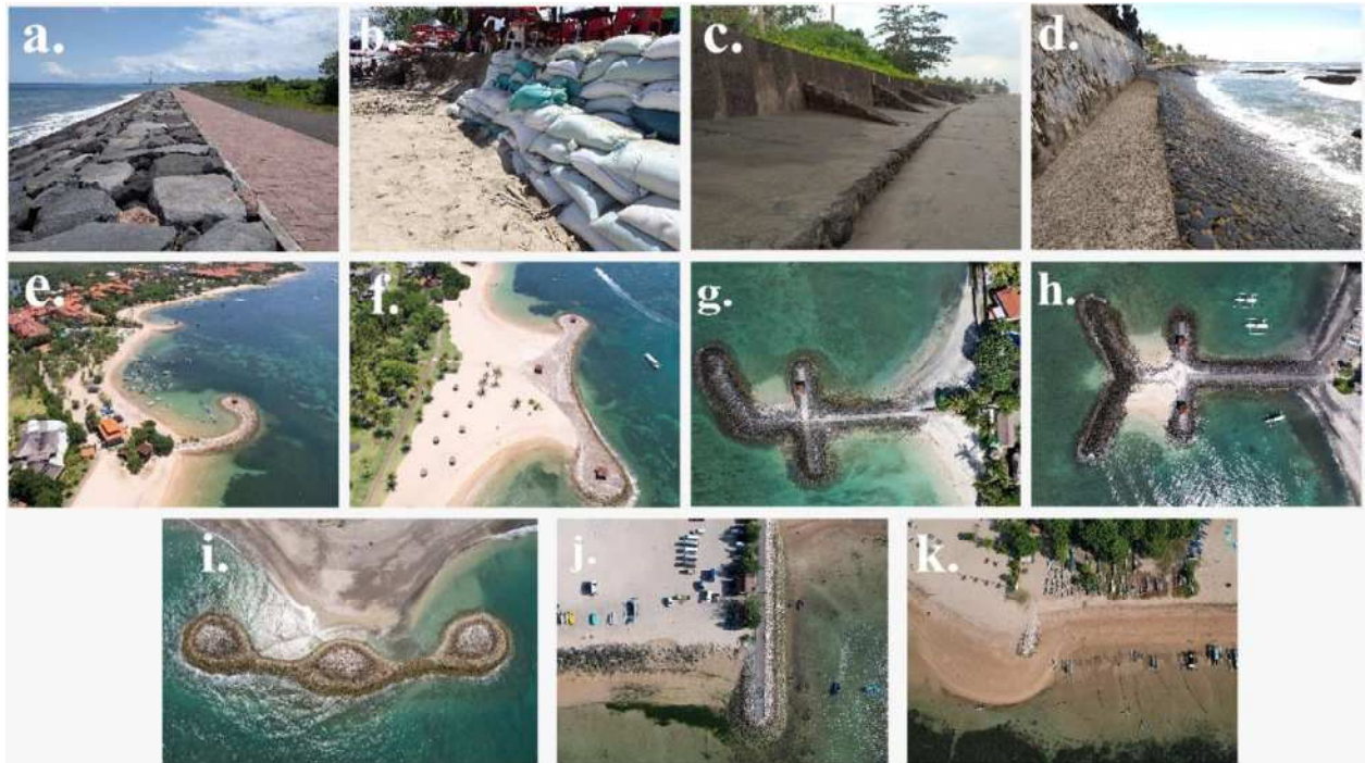
Figure 3-12. Various coastal protection structures in the study area: (a) Seawall with stone-filled gabions combined with revetment; (b) Sandbag at Kuta Beach, Badung Regency; (c) Seawall at Perancak Beach, Jembrana Regency; (d) Seawall at Pererenan Beach, Badung Regency; (e) Groins and (f) Offshore breakwater at Samuh Beach, Badung Regency; (g-h) Groins at Candidasa Beach, Karangasem Regency; (i) Offshore breakwaters at Jerman Beach, Badung Regency; (j-k) Groins at Sanur Beach, Denpasar City (Source: field survey, 10—19 March 2023).
