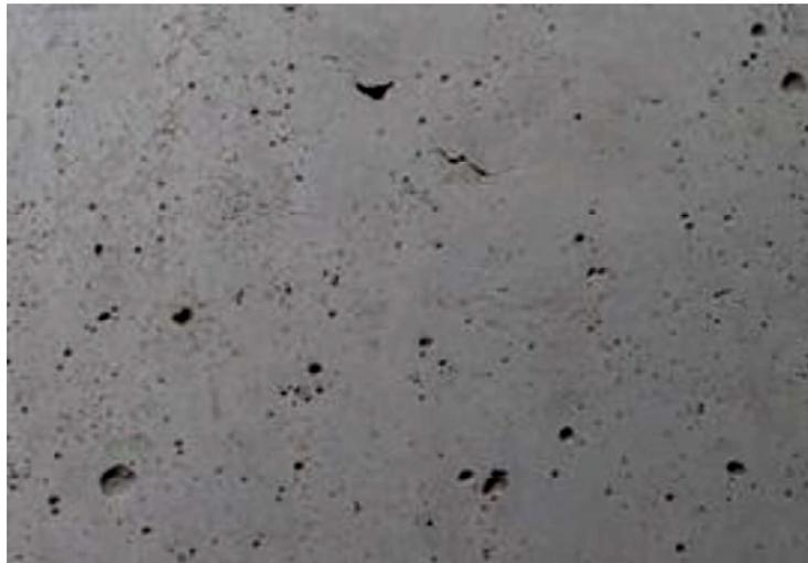
**Figure 2-2** Surface bugholes on the sidewall of tunnel lining concrete
