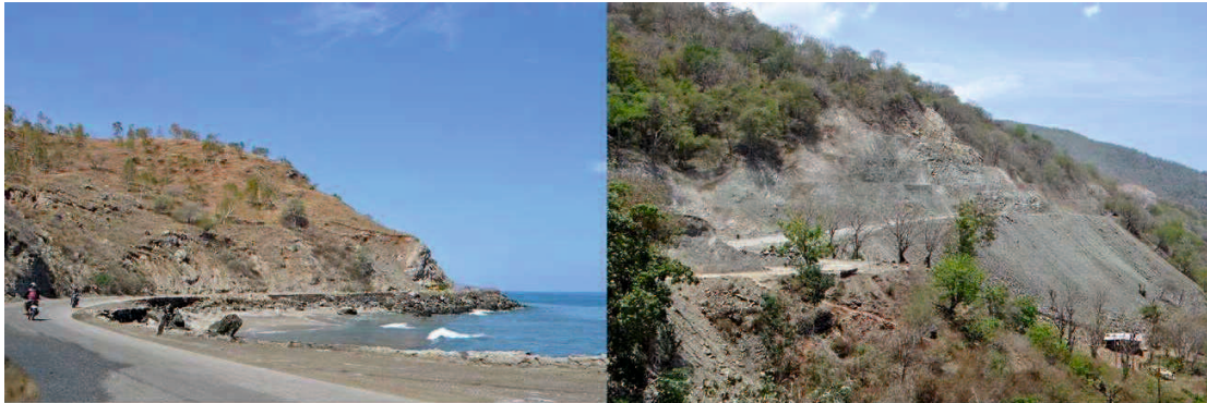
Old road condition
