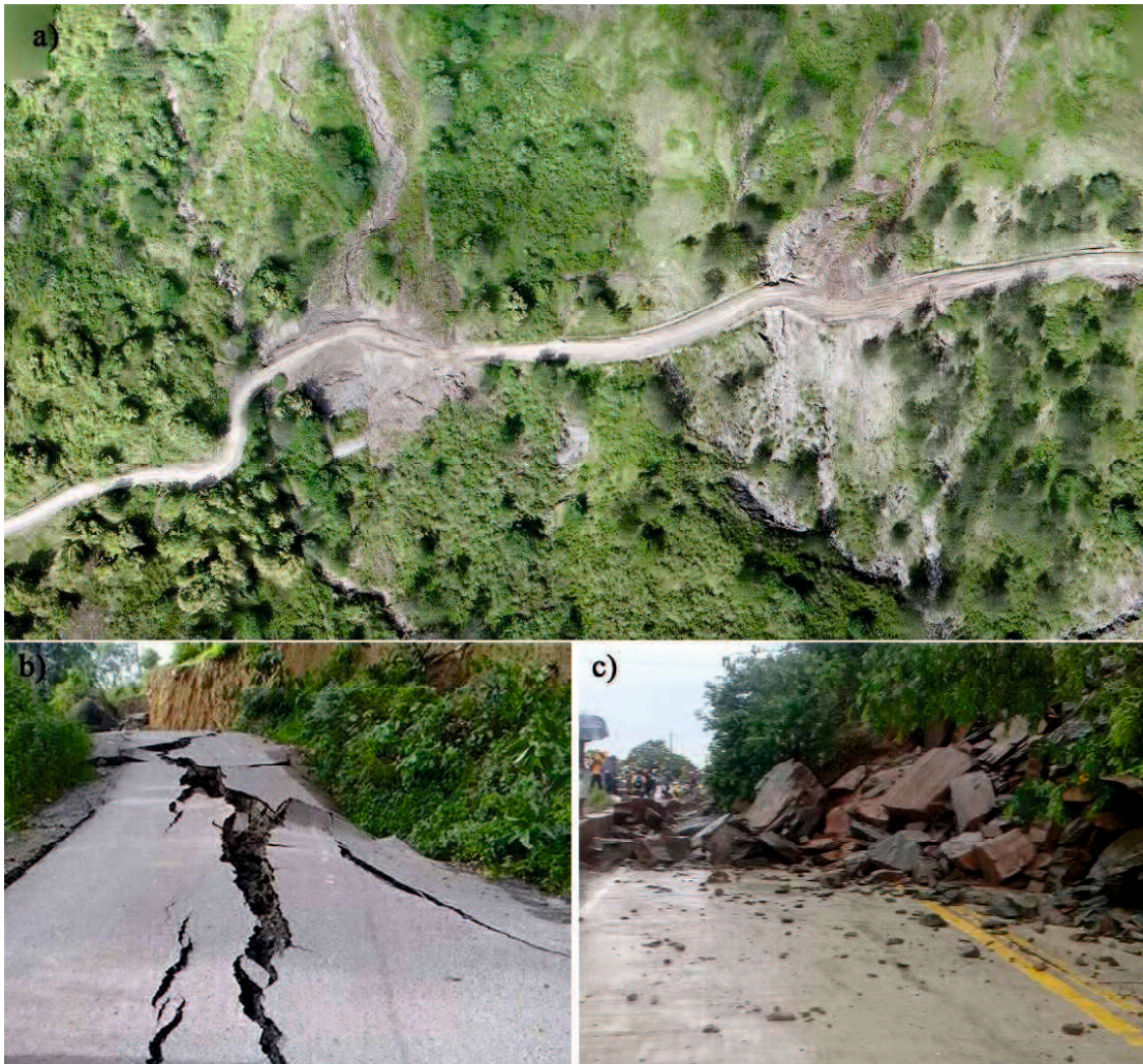
Figure 4.6. a) Aerial photo of Lekiatchi Landslide area, b) Landslide in Builico and affecting the road, photo by Biky , and c) Landslide in Batuboro and affected road, photo by Babo
