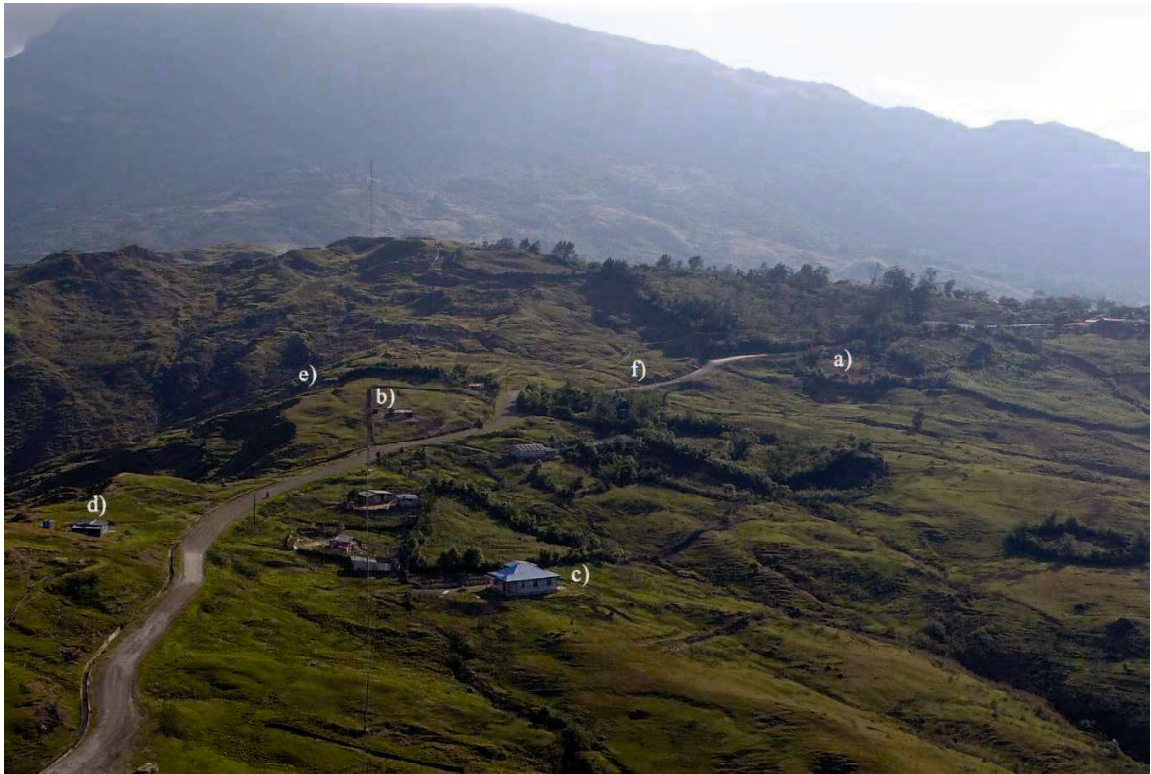
Figure 3.8. a) Location of house destroyed by a landslide in January 2017, b) New place chosen to build new house after January 2017 landslide, c) Expensive house built on unstable ground, d) House roof destroyed by a windstorm in February 2018, e) Landslide induced by an earthquake on 24 th June 2019, and f) Location of the study area related to the ground deformation
