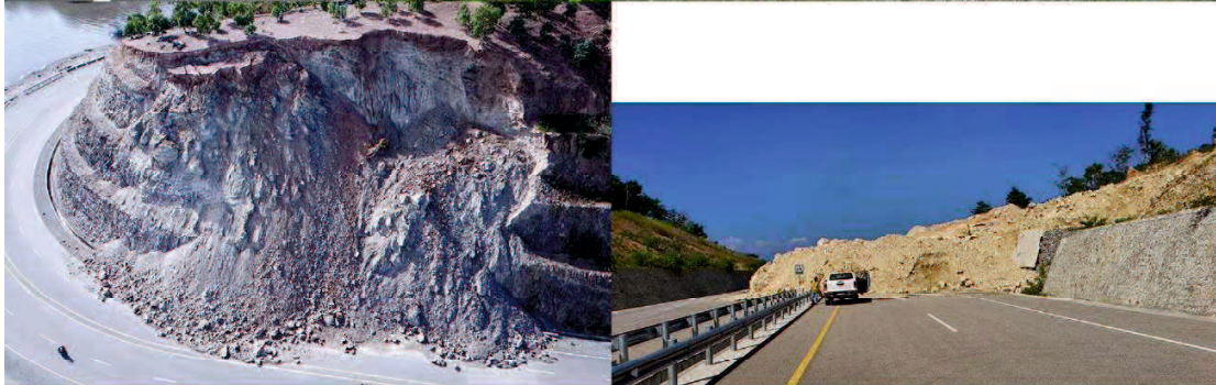
New road conditions
