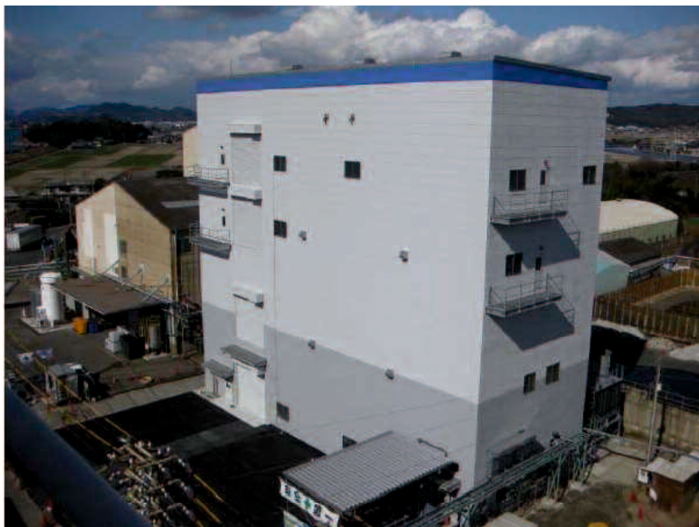
Fig. 5-1. Whole view of electrolyte plant.
