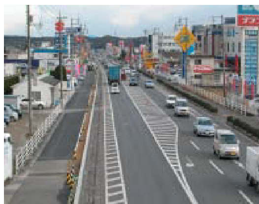
Photo 1 Overview of the road section
