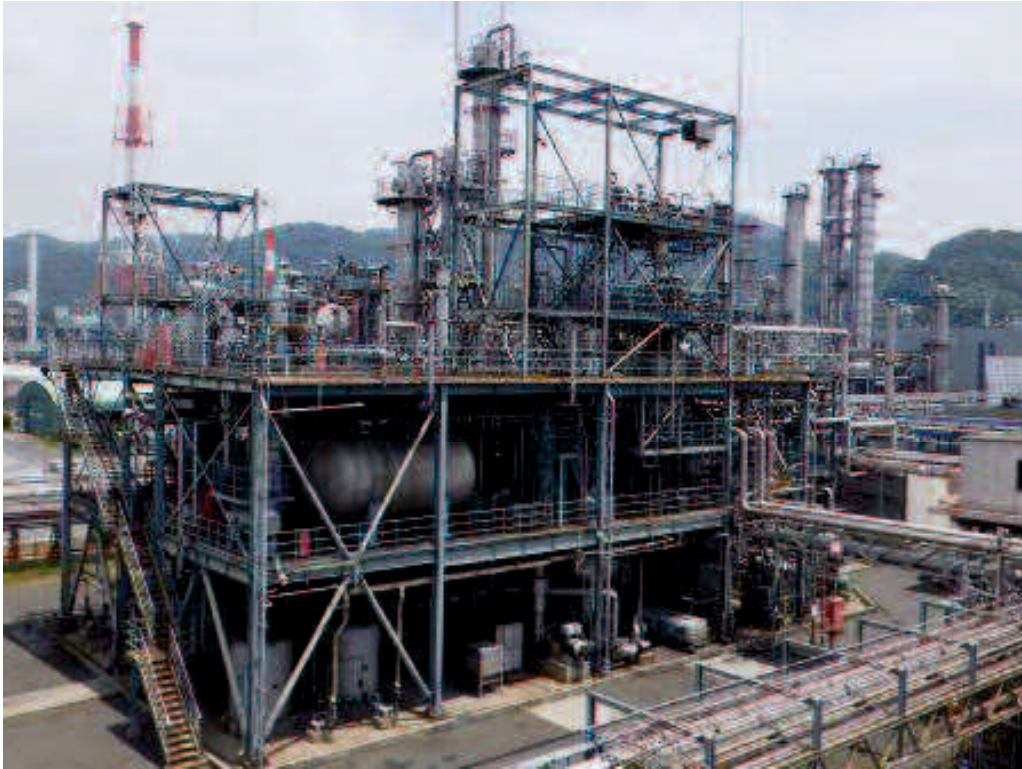
Fig. 5-1 Whole view of CPN plant
