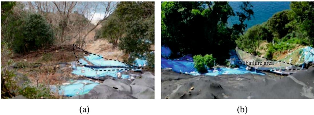
**Fig. 4.4.** Local failure around G1: (a) Situation on 28 January 2013 and (b) Situation on 31 August 2013 (adapted from Naya et al., 2014).
