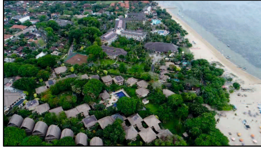
Figure 4.50 Field condition in the areas classified as damage zone of groundwater conservation with subsidence
