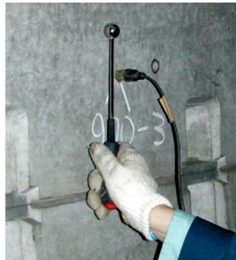
Fig.2.2 Inspection using an impact hammer 8) .
