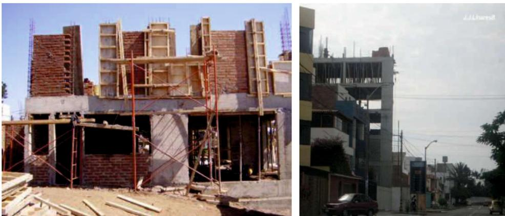
Figure 2.5 Typical non-engineered buildings in Puente Piedra, Carabayllo, Peru [Okazaki *et al.*, 2012]
