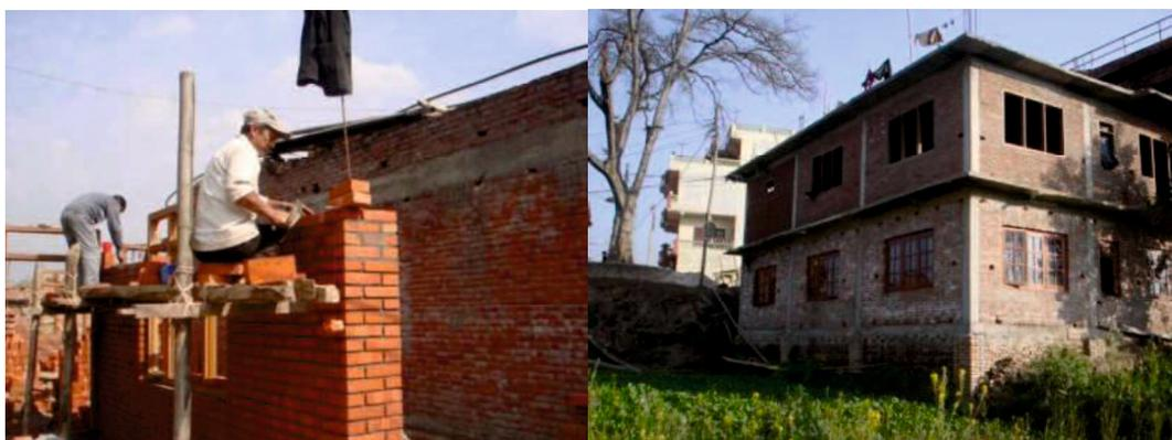
Figure 2.7 Typical non-engineered buildings in Balkot, Bhaktapur, Nepal
