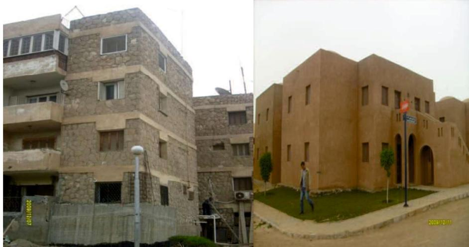
Figure 2.6 Typical non-engineered buildings in Egypt Helwan City, El-Marg City
