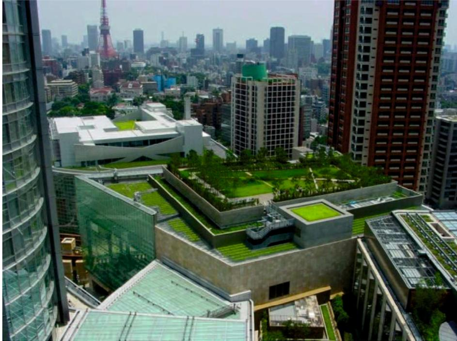
**Fig. 1-1.** Example of intensive green roof implementation.
