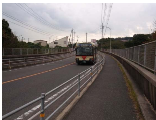
(c) 蛇瀬橋 (5径間橋)
