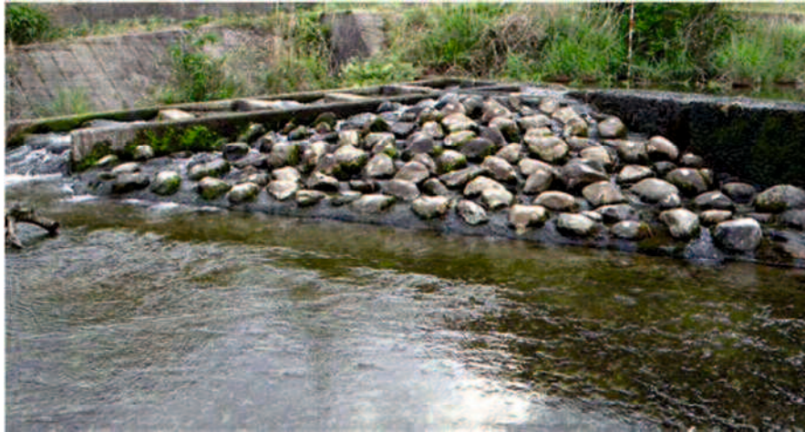
Fig. 5-1 Stone embedded on fish passage at Fushino River
