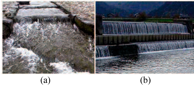
Fig. 4-1 Location of sounds recording. (a) Fish ladder in Misumi River; (b) weir of Fushino River.
