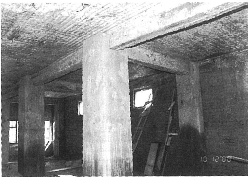
Photo. 3.63 Enlarged columns on the first and second story levels of the six-story hotel under construction at Biratnagar, Nepal
