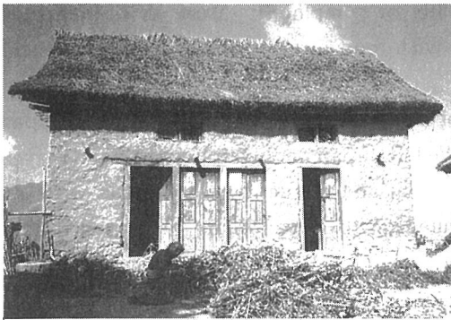
Photo. 1.1 Typical rural houses in Nepal (a) Mud-stone house in the Kathmandu Valley
