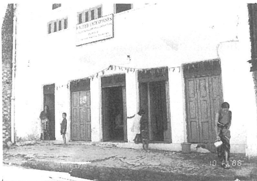
Photo. 3.57 An undamaged reinforced concrete private home; example 1, Dharan Bazaar, Nepal
