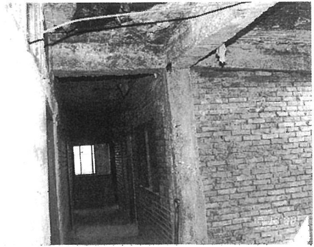
Photo. 3.62 Interior view of the six-story hotel under construction at Biratnagar, Nepal
