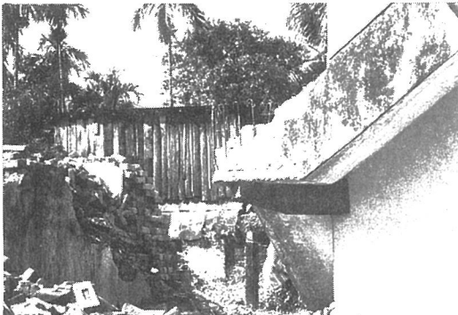
Photo. 3.55 The damaged two-story reinforced concrete medical office at Dharan Hospital, Dharan Bazaar, Nepal
