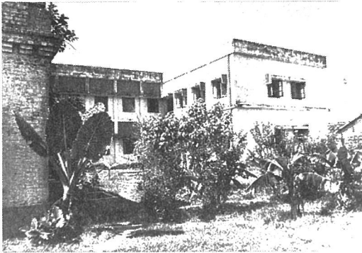
Photo. 3.51 An undamaged reinforced concrete building located next to the Civil Sergeant's Residence, Darbhanga District, Darbhanga, Nepal
