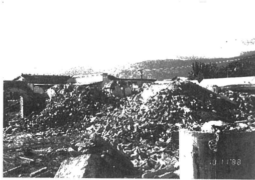
Photo. 3.42 The completely collapsed Dhankuta Hospital, Dhankuta Bazaar, Nepal
