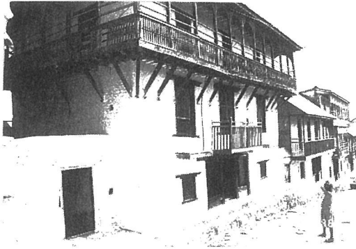
Photo. 3.40 Exterior view of a rural brick masonry house, Dhankuta Bazaar, Nepal
