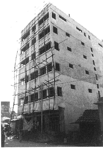
Photo. 3.61 Exterior view of the six-story hotel under construction at Biratnagar, Nepal
