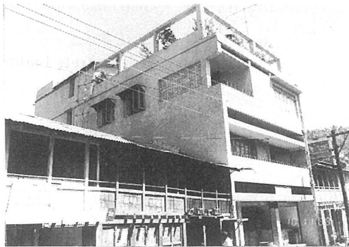
Photo. 3.58 An undamaged reinforced concrete private home; example 2, Dharan Bazaar, Nepal
