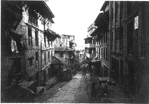
Photo. 3.22 Damage zone in the old town, Bhaktapur
