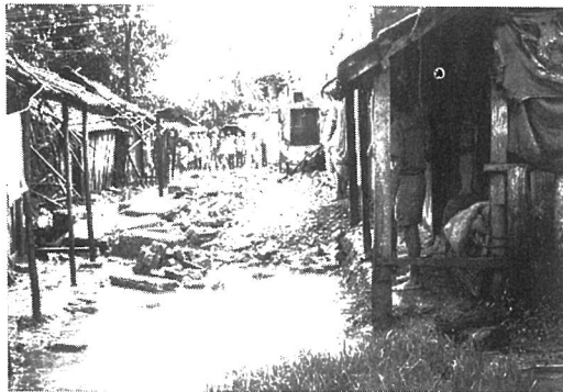
Photo. 3.43 A collapsed single-story brick masonry house in Biratnagar, Nepal (photo taken by a resident just after the shock)
