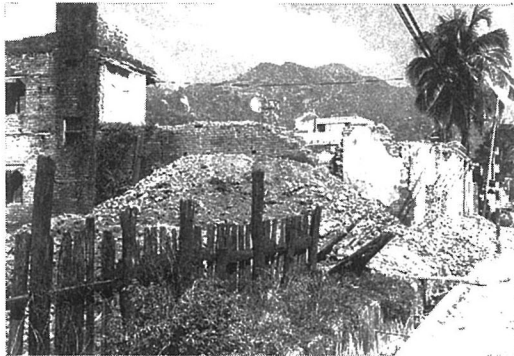
Photo. 3.30 A collapsed brick masonry house; example 2, Dharan Bazaar, Nepal
