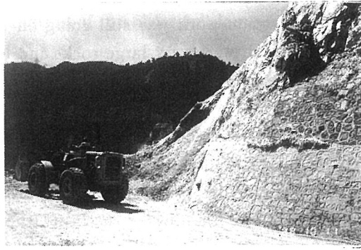
Photo. 3.69 Rockslide site undergoing restoration
