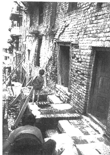
Photo. 3.25 The expanded wall of a brick masonry building, Bhaktapur, Nepal
