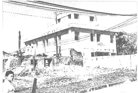
Photo. 3.56 The telecommunications office, Dharan Bazaar, Nepal
