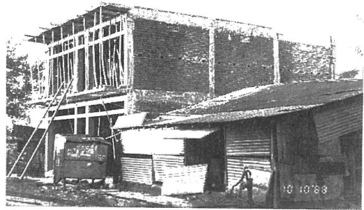
Photo. 3.48 A reinforced concrete building under construction in Biratnagar, Nepal
