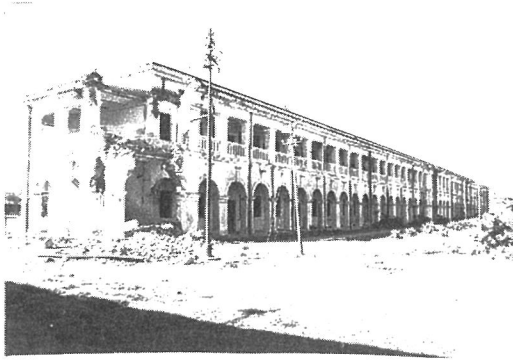
Photo. 3.17 The damaged Medical College Hospital, Darbhanga
