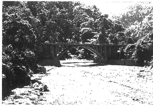
Photo. 3.68 Undamaged arch bridge
