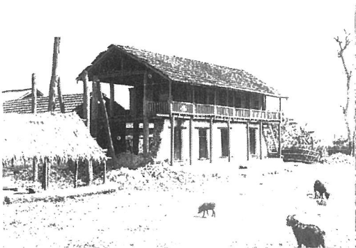
Photo. 3.26 A damaged brick masonry farm house, Gaighat, Nepal
