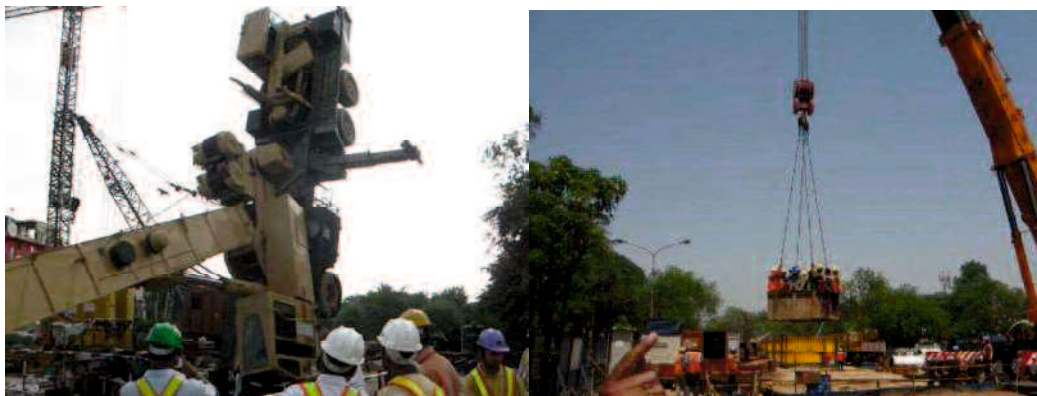
Photo 5-9 Poor safety condition at a construction site in India
