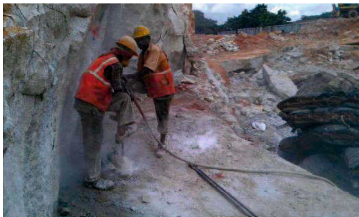
Photo 1-2 Drilling work at the Indian Metro construction site
