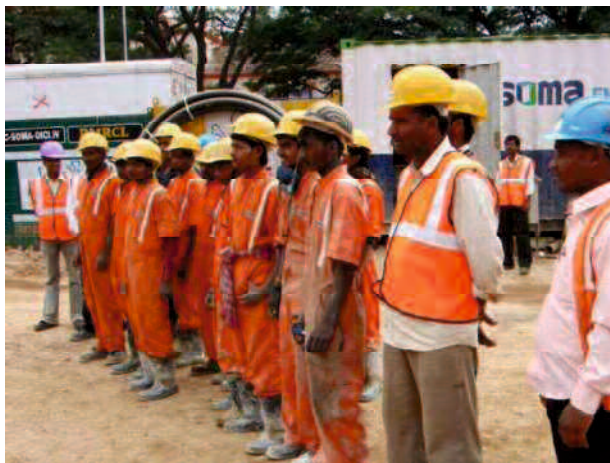
Photo 5-7 Environmental training by the contractor at the Bangalore Metro site
