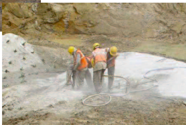
(b) Drilling work
