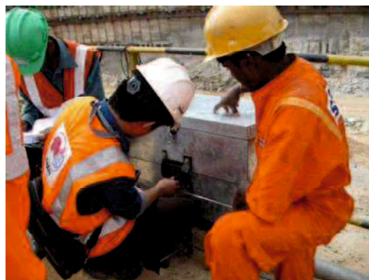
Photo 3-4 Dust monitoring system consisting of chassis box with mobile phone camera
