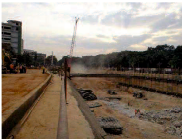
Photo 1-1 Construction site of the Indian Metro Project
