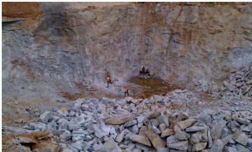
Photo 2-7 Environmental condition at a construction site in India
