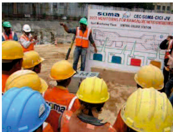
Photo 5-5 Environmental training at the Bangalore Metro construction site
