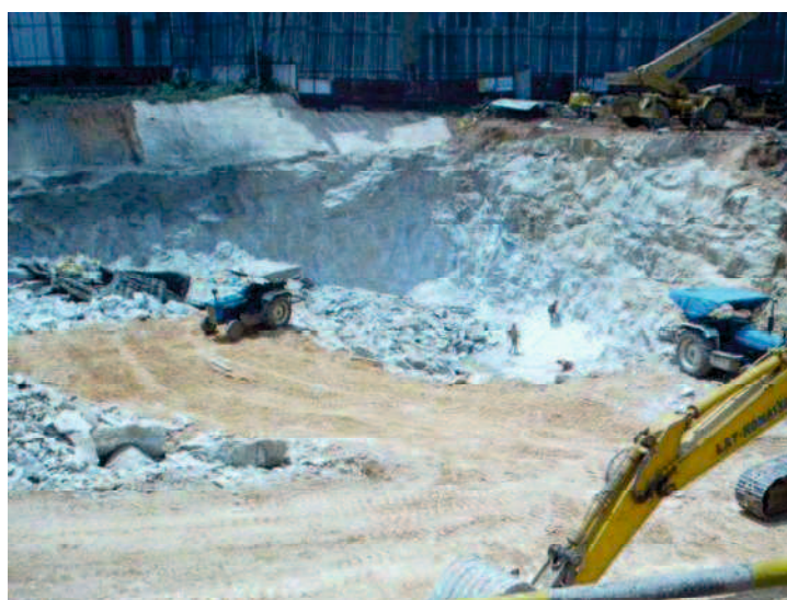
Photo 2-1 Drilling and blasting work at the Indian Metro station site
