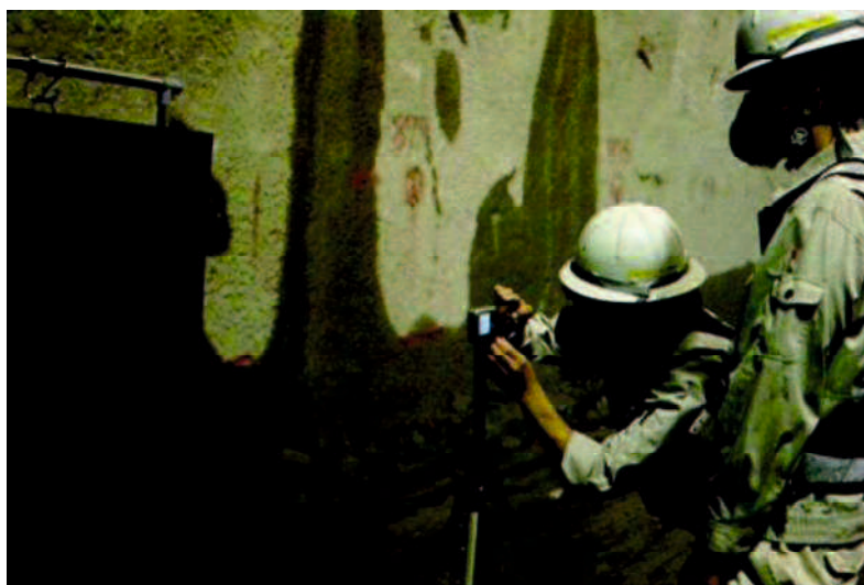
Photo 3-2 Black panel installation
