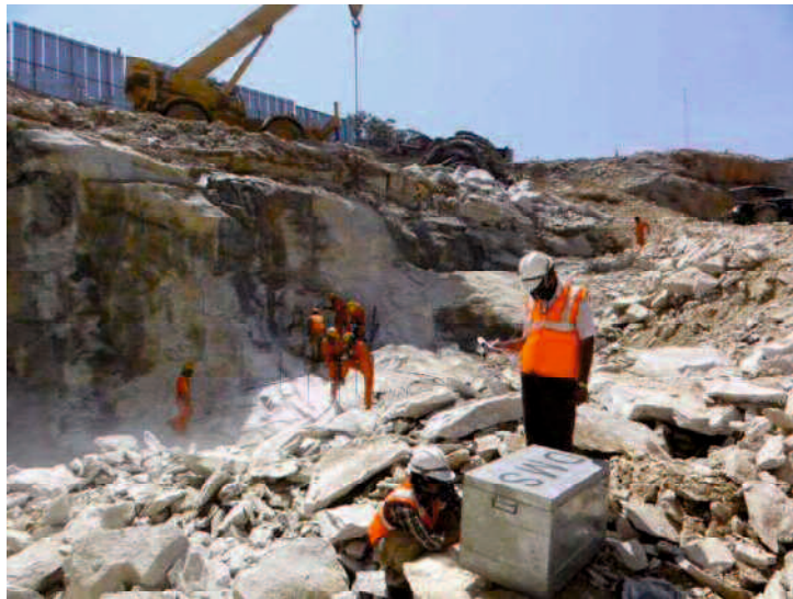
Photo 4-1 Dust monitoring box at the open excavation site
