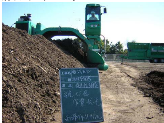
Photo 3. The work scenery of the intermixing.
