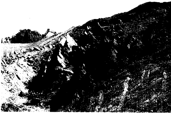
Photo. 3 The state of saw failure of slope I
