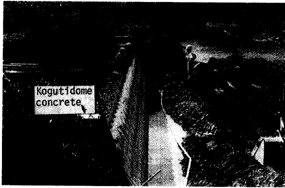
Photo.1 An example of "Kogutidome-kou" used in river improvement
