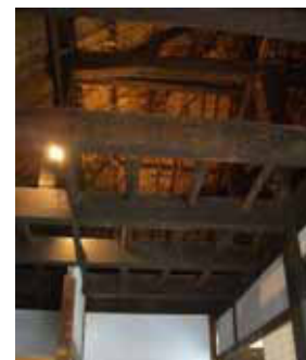
Photo.9 Interior of Doma (H17)
