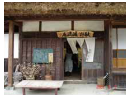
Photo.10 Exterior of Entrance (H17)
