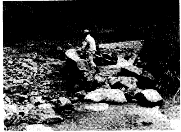
Photograph E Side erosion near the downstream end of revetment (Hieda river)
